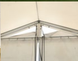
Gable vents with adjustable cover flaps
