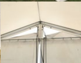
Gable vents with adjustable cover flaps
