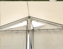
Gable vents with adjustable cover flaps
