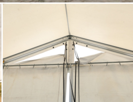
Gable vents with adjustable cover flaps
