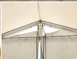
Gable vents with adjustable cover flaps
