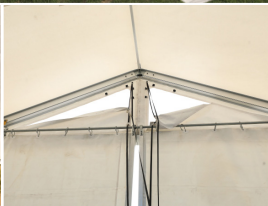
Gable vents with adjustable cover flaps
