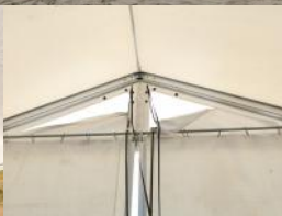
Gable vents with adjustable cover flaps
