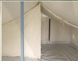
Inner tent to provide insulation, humidity control, and privacy.
