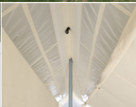
Ventilation windows along the ridge line.
