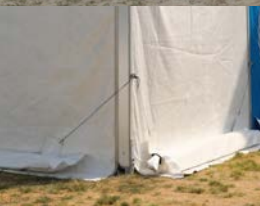
Ballast anchors (to be filled with sand, stones or water)
