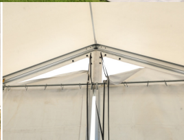
Gable vents with adjustable cover flaps
