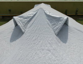
4 roof vents to provide full airflow from all direction.
